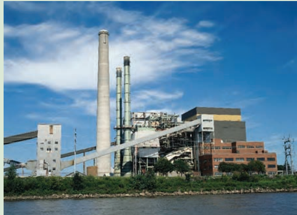
Ohio Edison plants provide electrical service to more than 1 million customers. © Don Farrall Getty Images/PhotoDisc.
